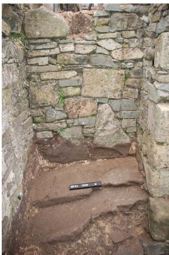
Plate 2: Area 1, sandstone walkway slabs (1004), view W
