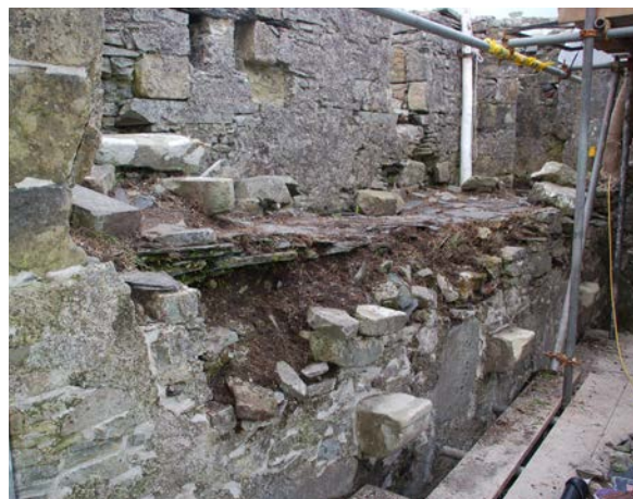
Plate 8: Area 6, corbels for longitudinal beam, view NW
