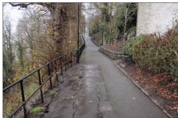
Plate 2: Damage to the Back Walk prior to reconstruction.
