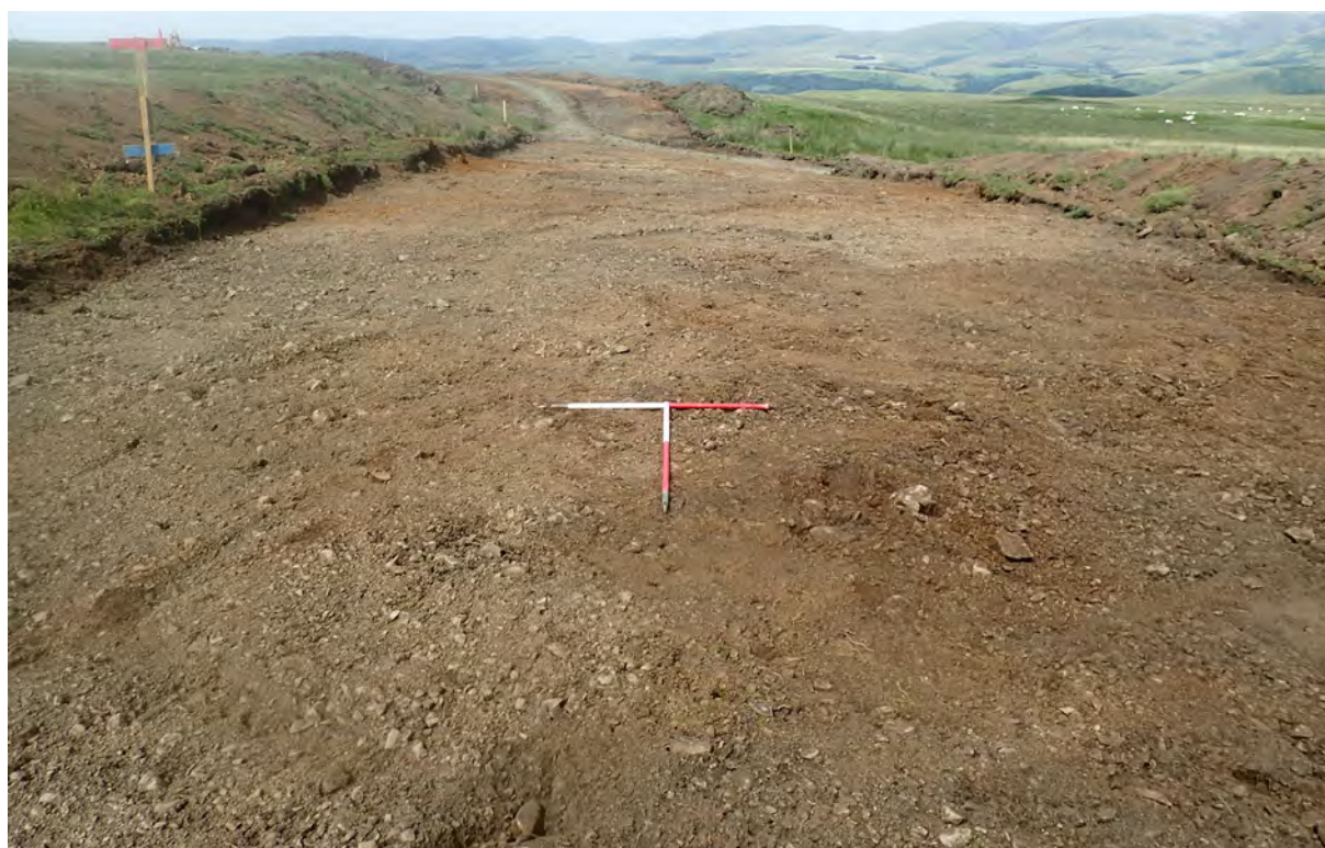
Figure 2: The wind farm route stripped of topsoil.
