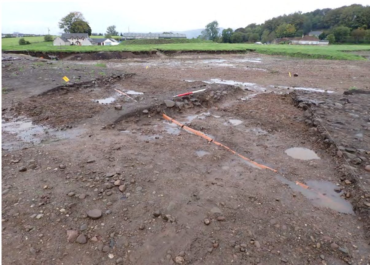
Figure 15: Slot 3 after removal of road (003) along the course of the proposed housing development's spinal road, from the south-west.
